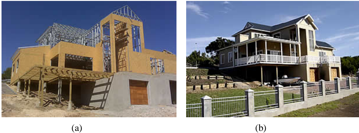
Figure 1. Steel frame under fabrication and a completed house on a slope.
