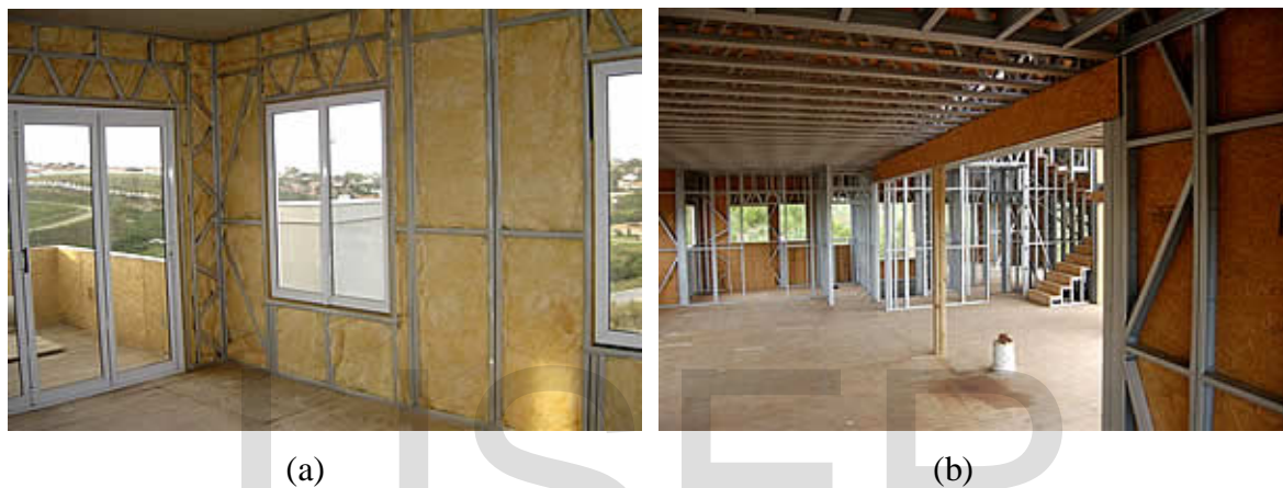
Figure 2. Panels used as walls.
